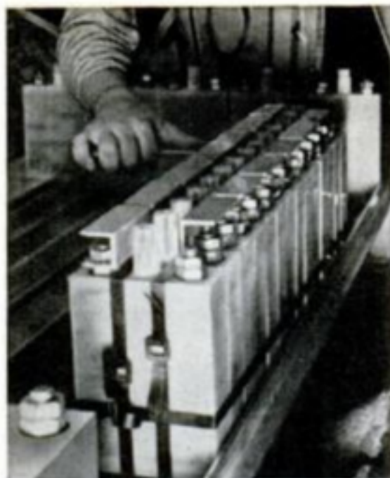
NICKEL-CADMIUM cells, rated 75 ampere-hours each, are installed
